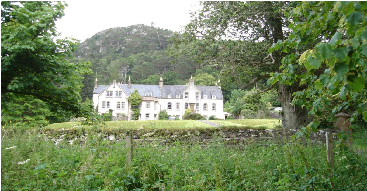
Flowerdale House, Gairloch. Built 1738 by Alexander MacKenzie, 2 nd Bart.
